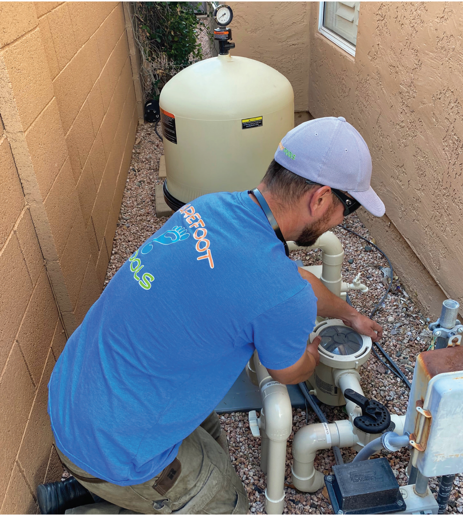
Garcia swaps out a pump in a tight space.
